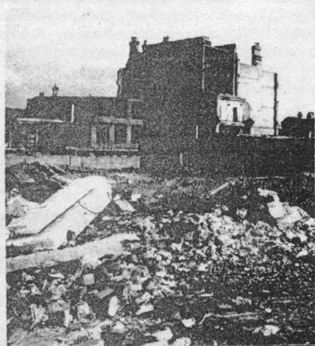
All that was left of the Eddystone works after the November, 1948, bombing - the event which caused the move to 'The Bath Tub'
